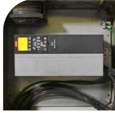
Installation of VFDs in Our Motors to Control the Cooling Tower
