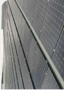
Installation of Canteen Solar Roofing
